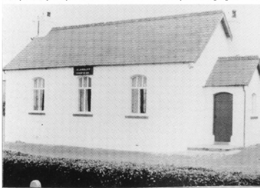
The school which was erected in 1899.
